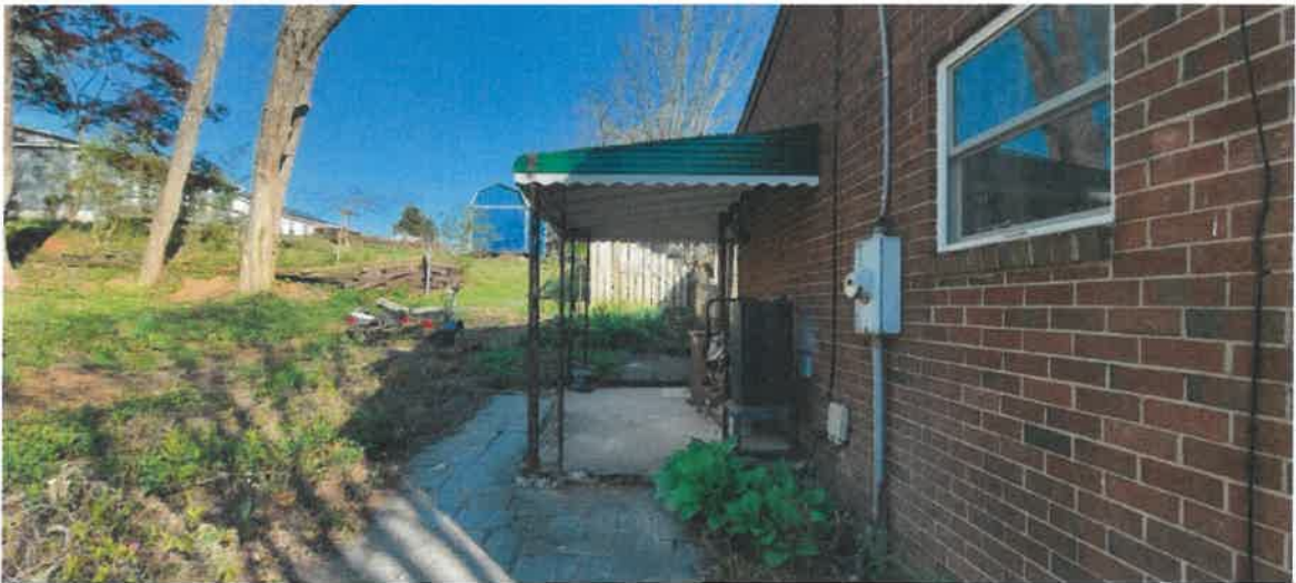
View of side patio and awning facing east from driveway.
