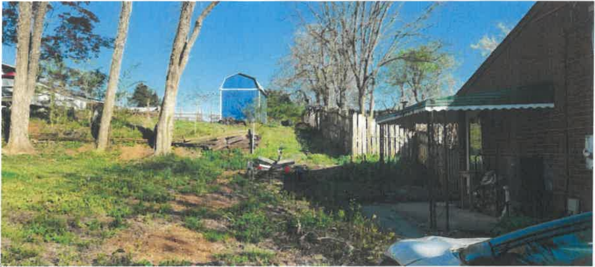
View of side patio and awning from Rialto St. facing east.
